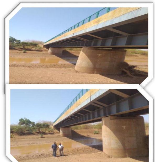
Figure. 9:- constructed bridge by Poly GCI
