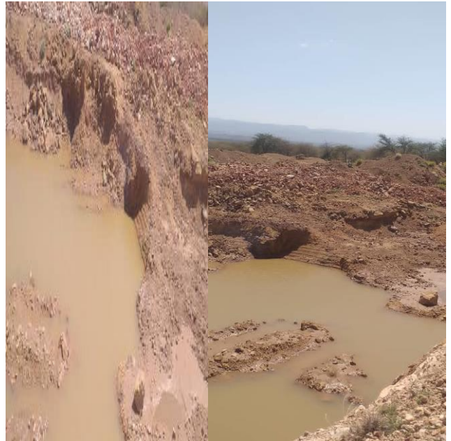
Picture 1. Opening pits with unsafe water
